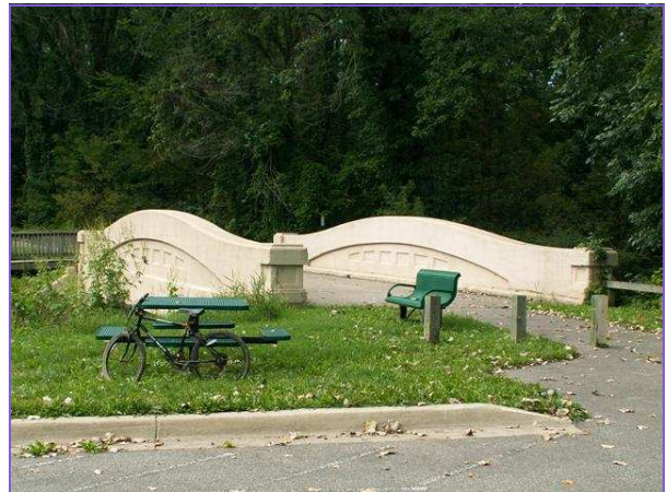
Mill Road Bridge
